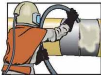
4. Blast clean surfaces to a near white ISO-8501, NACE No. 2, SA-21/2 (SSPC-SP 10) or better using particle blasting (sand or other). Sweep blast adjacent FBE or CTE coating. 50 mm (2") to either side of cutback (the bare steel area)
