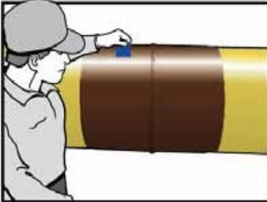
11. Use a Wet Film gauge to measure that the desired minimum thickness has been achieved. Double check around the weld to insure minimum desired thickness.
